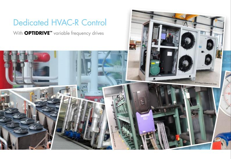
Installation of **OPTIDRIVE<sup>™</sup>** variable frequency drives to control refrigeration compressors, significantly reducing energy consumption, and improving system COP (coefficient of performance)
