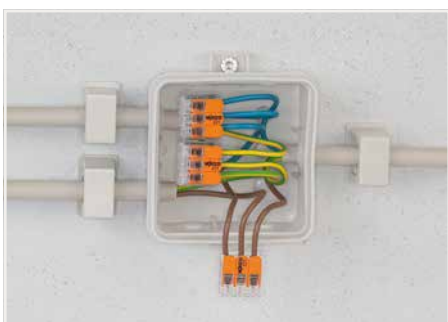
Wiring fine-stranded conductors in a junction box.
