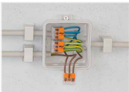
Wiring fine-stranded conductors in a junction box.
