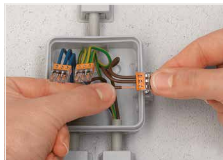
Insert the stripped solid conductor until it hits backstop.
