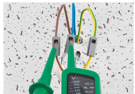
Testing via separate test ports.
