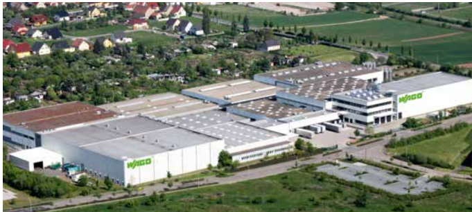
WAGO Sondershausen, Germany
