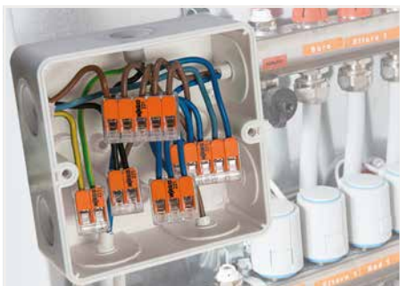
Wiring fine-stranded conductors in a junction box.
