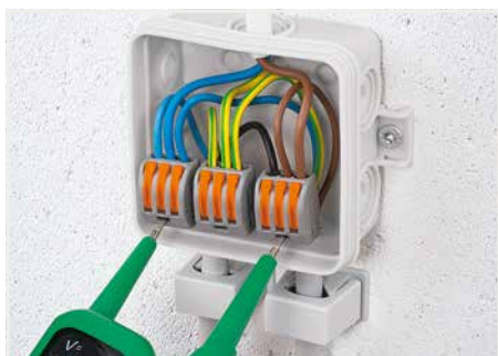
Testing the wired connectors
