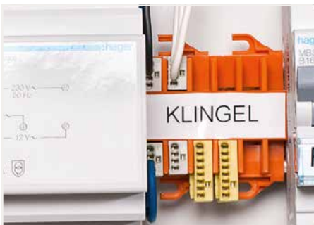
DIN-35 rail-mount application (residential door bell)
