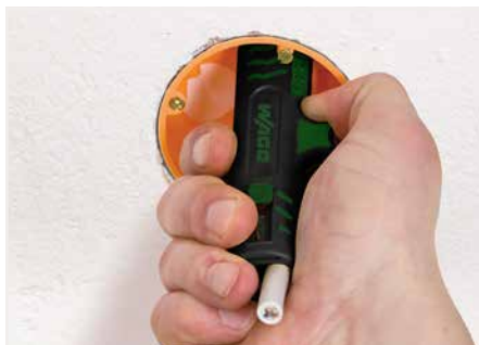
Stripping a cable sheath.
