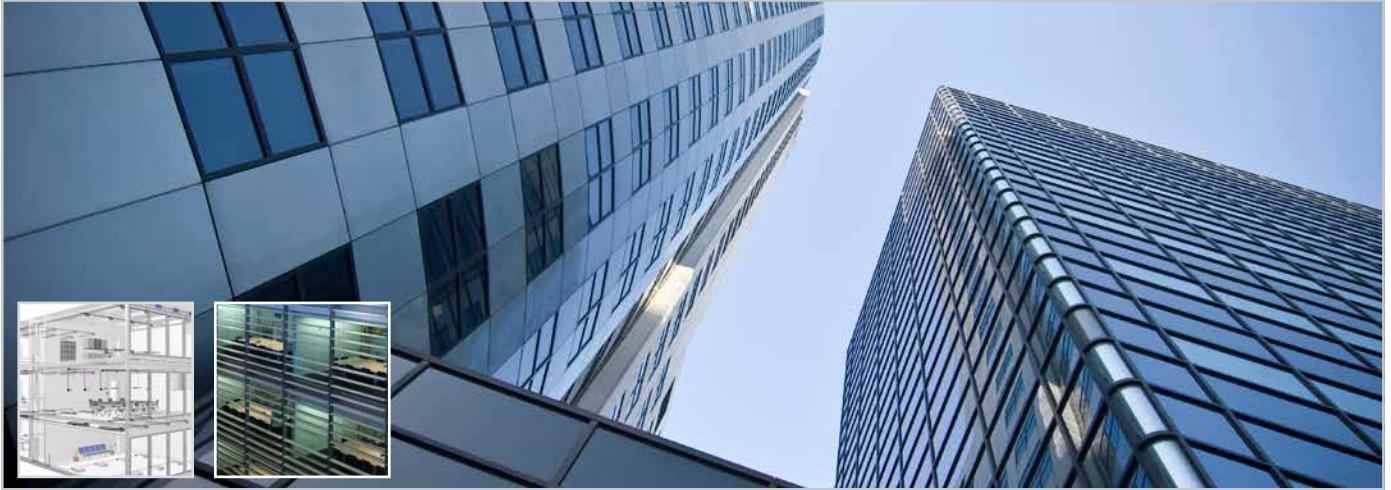
Building installation and automation
