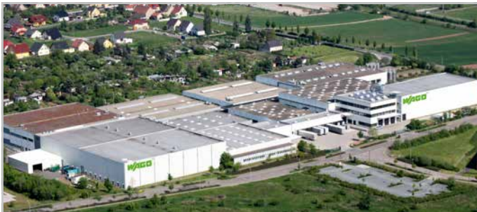
WAGO Sondershausen, Germany
