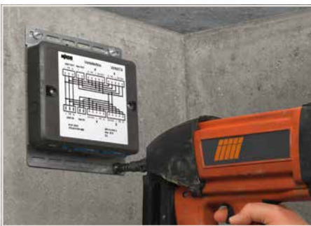
Securing the mounting plate with WINSTA® Distribution Box to the wall (e.g., via stud gun).
